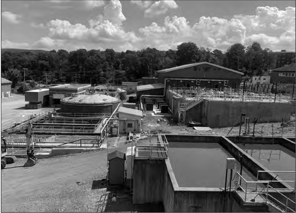
Figure 1. The Penn State's Wastewater Treatment Plant (photo by M. Smol, August 2022)
