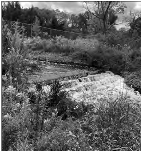
Figure 4. Water discharged from the University Area Joint Authority to a natural reservoir (photo by M. Smol, August 2022)
