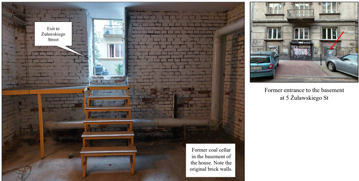
Fig. 17. Possible location of HeChalutz HaLochem's command centre in a basement at Żuławskiego 5 in 1942, photos by Eran Zohar, September 2024
